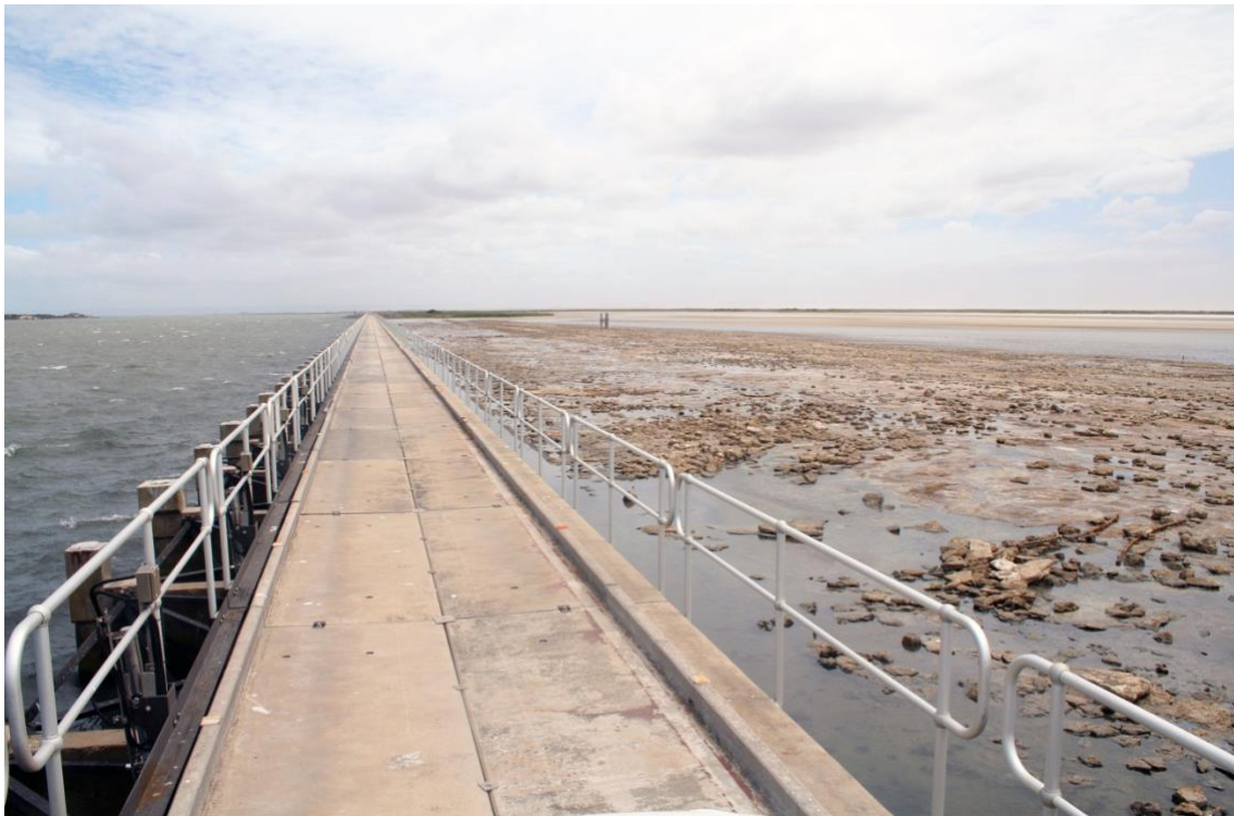
Fig 55: Bonita Ely (2009) Barrage #4: The Coorong Meets Lake Alexandrina. Barrages hold back the ocean and the Coorong (left) from flooding Lake Alexandrina with saline water. January, 2009.
