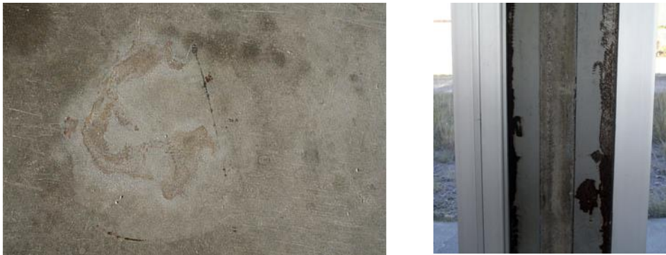
Fig 22: (Left) The stained concrete floor in Judd's sheds, Marfa Texas. (Right) The window frames show exposed applications of glue. Photo. B. Ely, 2008.
