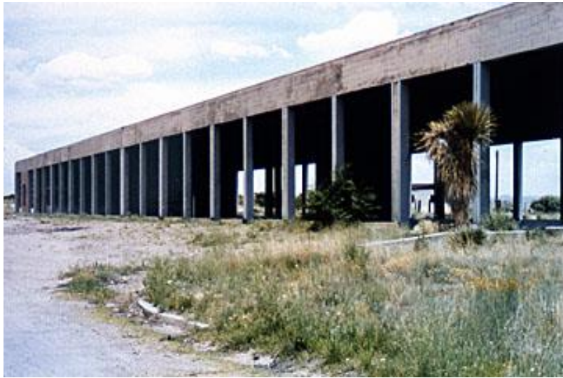
Fig 13: Judd's renovation of the Fort Russell artillery sheds in progress.
