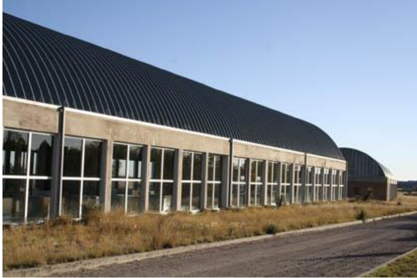
Fig 15: The two gun sheds showing the squared aluminium windows and off set alignment. Photo. B. Ely, 2008.
